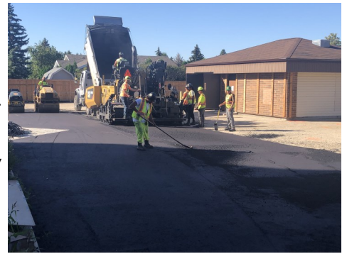
Paving, South Staff Parking Lot
